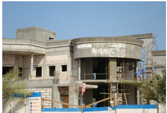
Photo 3 (left): Under the Las Vegas stucco. Wood frame (2×6) externally insulated with expanded polystyrene installed over a drainage plane. Thermal resistance is nominally R-25. Tile roof is installed over unvented conditioned wood frame insulated assembly. Thermal resistance is nominally R-35. Photo 4 (right): Under the Dubai stucco. Concrete masonry units are not insulated. Thermal resistance is nominally R-8. The roof membrane is installed over an unvented, uninsulated conditioned concrete slab. Thermal resistance is nominally R-8.
