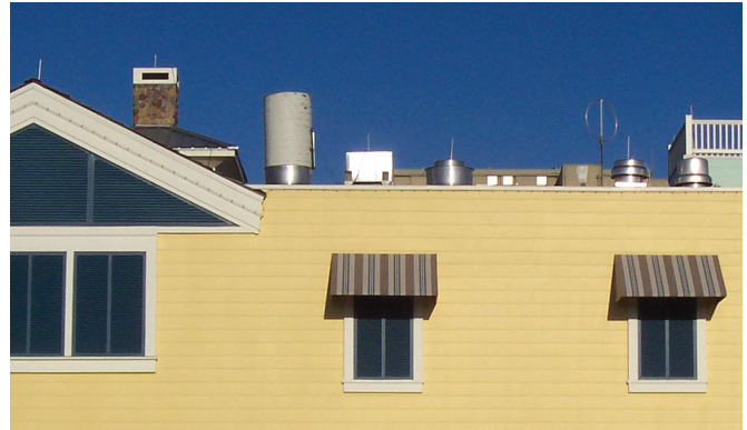
Photo 1 (left): Low velocity laminar flow replacement air outlet. Photo 2 (right): Stack extension on an upblast power roof ventilator.
